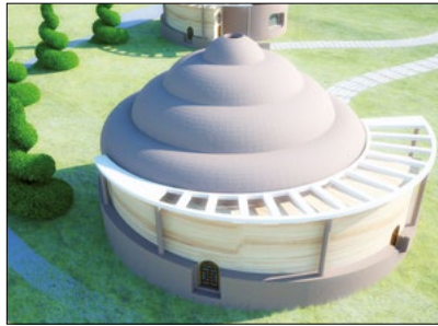
The organic forms of Djanan's architecture are to be created predominantly in earth bag construction. Nylon bags are suspended in a frame at 20 cm intervals, filled with clay from above and then pressed tight. Clay as well as raffia or wire mesh are also used for the upper plaster – all of them inexpensive materials. © all pictures by Kautz-Vella
